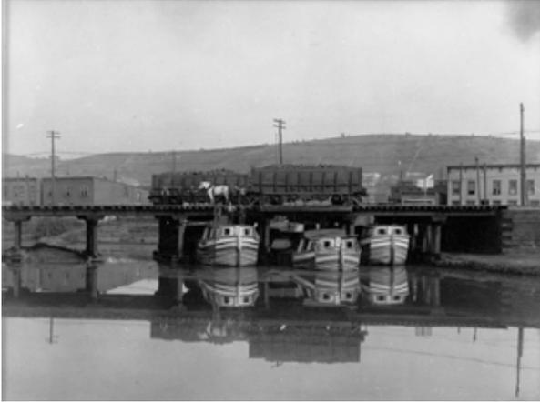
Canal boats being loaded with coal via rail bridge at Cumberland, MD. Note the difference in freeboard between the loaded and unloaded boats. (Special Collections Research Center GWU)
