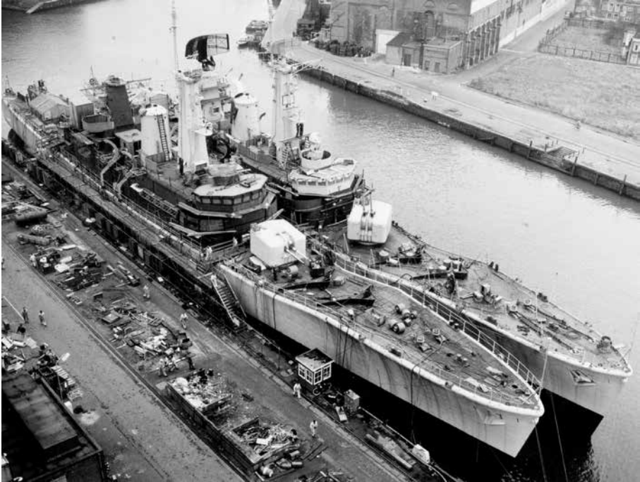
Van Speijk-class frigates Van Nes and Van Galen under construction in 1966. (Wikimedia Commons)
