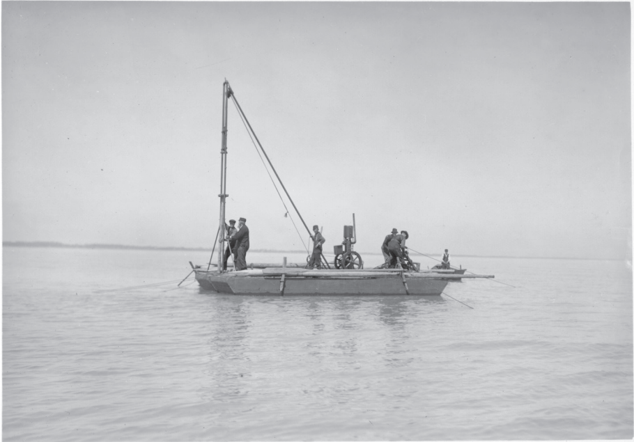
Suction dredge on the St. Clair River, [1911]. (John Boyd, photographer. C 7-3-0-680, John Boyd fonds, Archives of Ontario)
