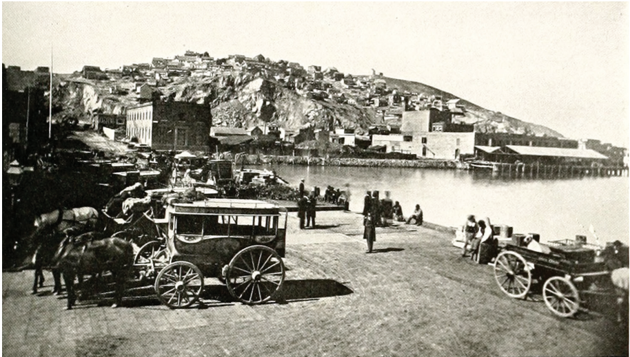
An Early Wharf, c. 1860, with Telegraph Hill in the background. C.L. Hill and C.A. Kofoid, eds., Marine Borers and Their Relation to Marine Construction on the Pacific Coast: Being the Final Report of the San Francisco Bay Marine Piling Committee (Published by the Committee, 1927), 17.
