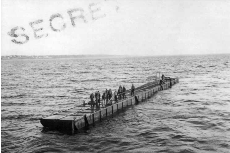
An assembled 2X30 pontoon causeway section. (Image provided by Andrew Hussey, Manston, UK)
