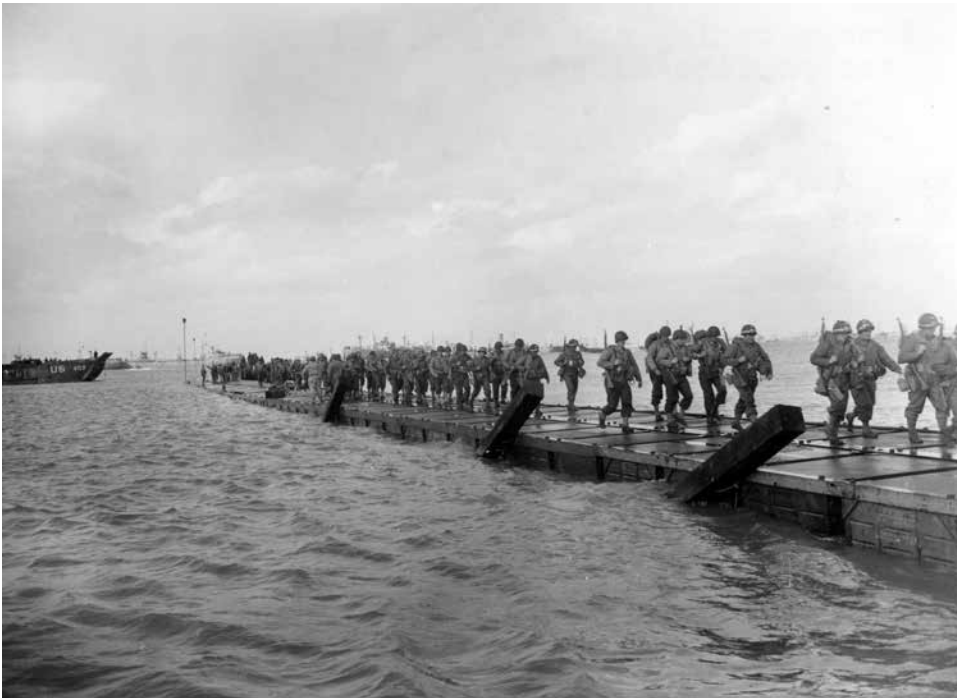
Soldiers marching ashore across pontoon causeways, most likely at Utah Beach. (US Navy Seabee Museum, Port Hueneme, CA)
