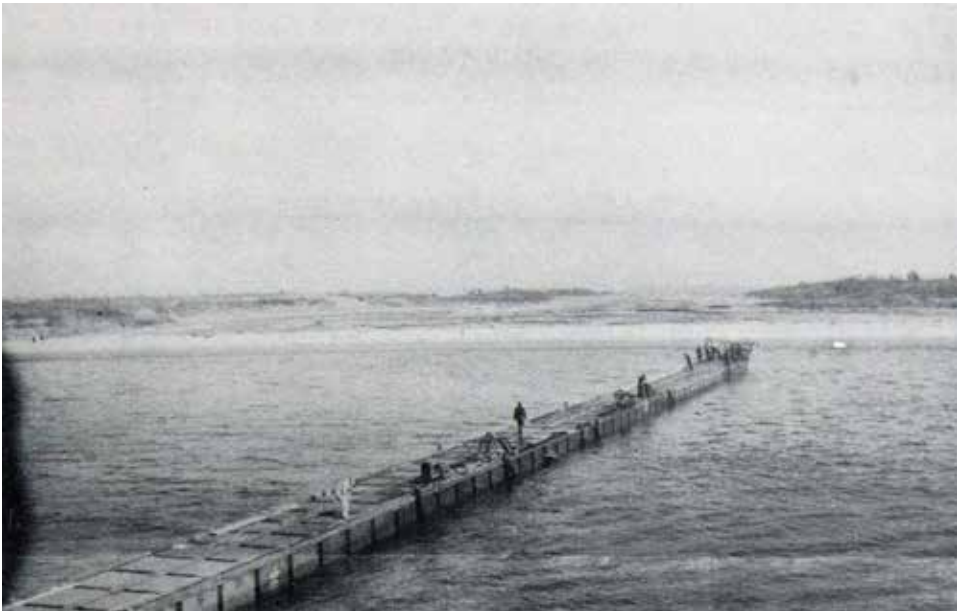
Assembled pontoon causeway at Narragansett Bay, 18 March 1943. (Bureau of Yards and Docks, Handbook on the Use of N.L. Pontoon Causeways and Army Steel Treadway Pontoon Bridges for Ship-to-Shore Connections Between LST Ships and a Gently Sloping Beach (Washington, DC: Navy Department, April 1943), 30)
