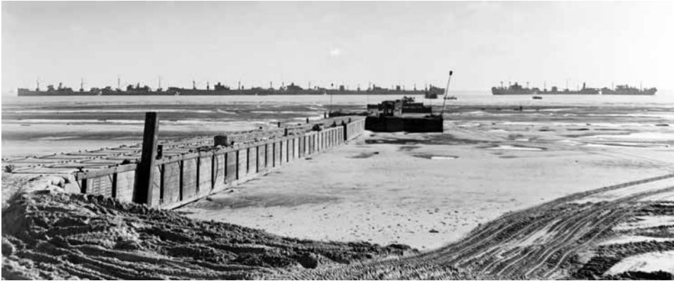
Causeway No. 2 at Omaha Beach at low tide with blisters visible, 12 June 1944. Part of the gooseberry breakwater of Mulberry A can be seen in the background. (National Archives and Records Administration)
