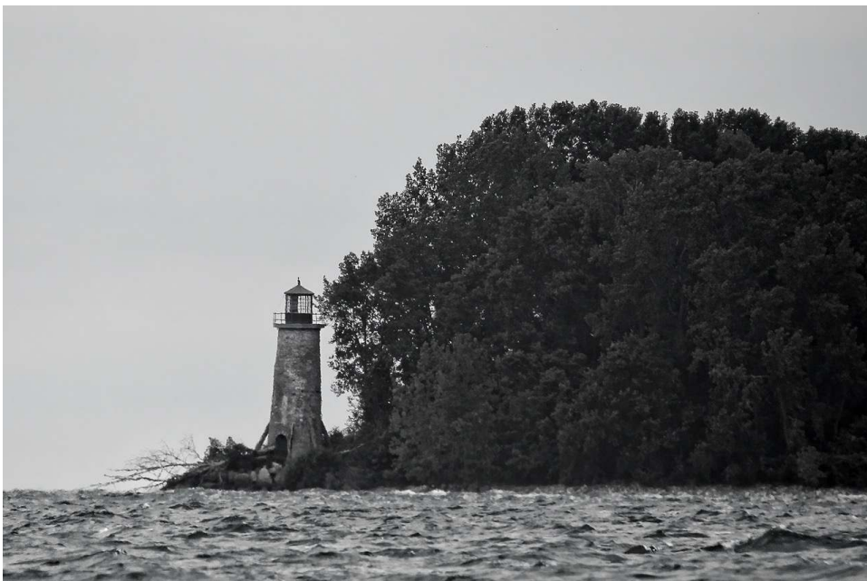
The 1833 Pelee Island light still stands, thanks largely to the heavy timbers propping it up at the base. It was decommissioned in 1909, but substantially restored by 2000. Photo by Diane Bédard.
