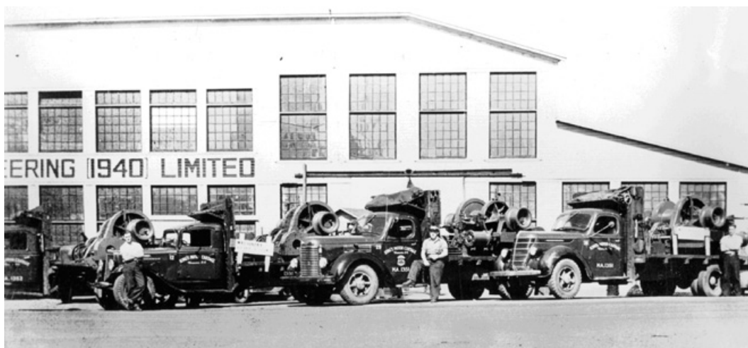
Illustration 5: Windlasses manufactured by Heaps Engineering (1940) Limited loaded onto flatbed trucks for delivery to nearby Vancouver shipyards to meet progress schedules. Wartime saw more extensive use of sub-contracting to industrial firms and pre-fabrication of components in British Columbia's Lower Mainland. (New Westminster Public Library)
