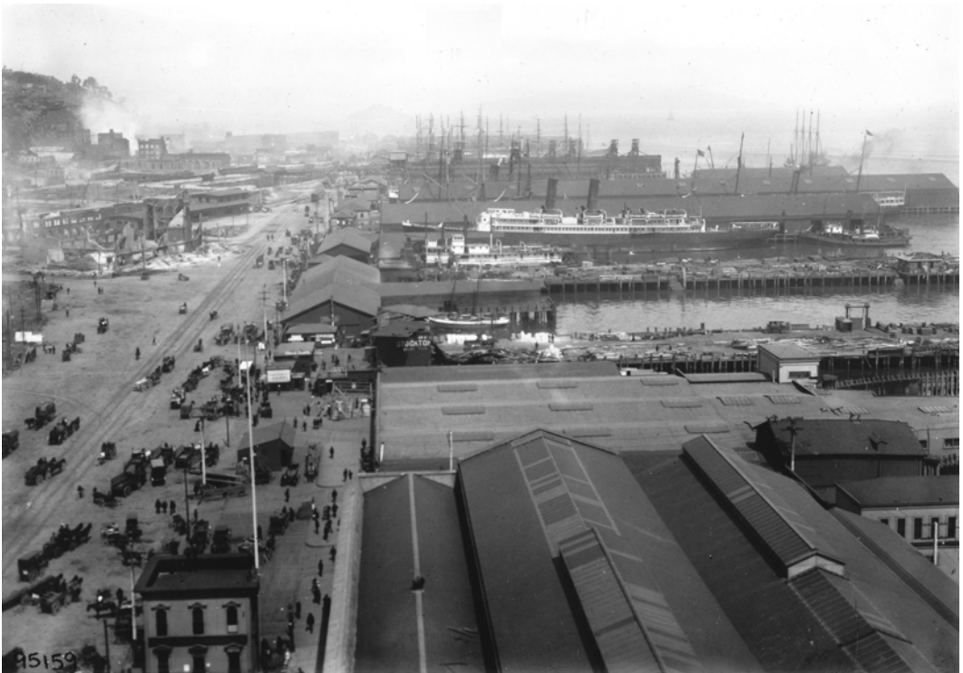
Fig 4: San Francisco Waterfront—This photo is taken from the Union Ferry Building looking towards Telegraph Hill. (National Archives)
