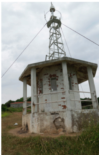
Watch tower base
