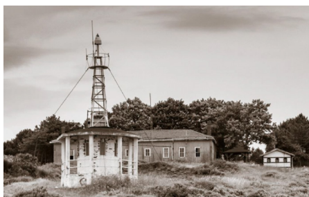
Watch tower base with refuge house behind
