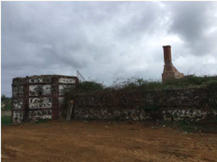
Watch tower base, with chimney of mansion within the walled enclosure
