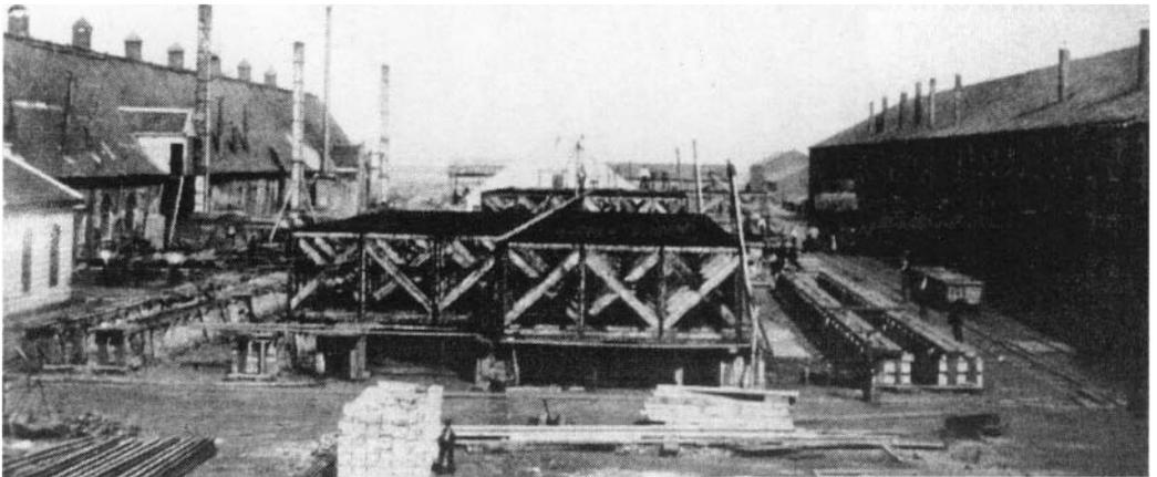
*Figure 3:* The drydock in construction at the Royal Factory of Paul van Vlissingen and Dudok van Heel in Amsterdam, c. 1863.
