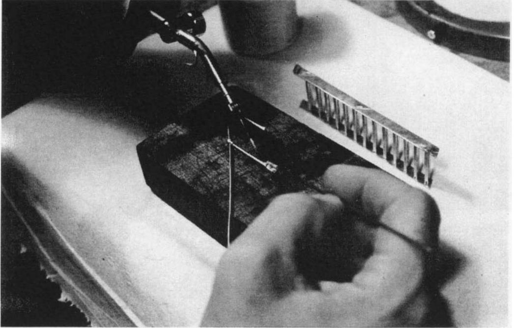
*Figure 13:* Hard soldering is done with a hydrogen flame and silver.
