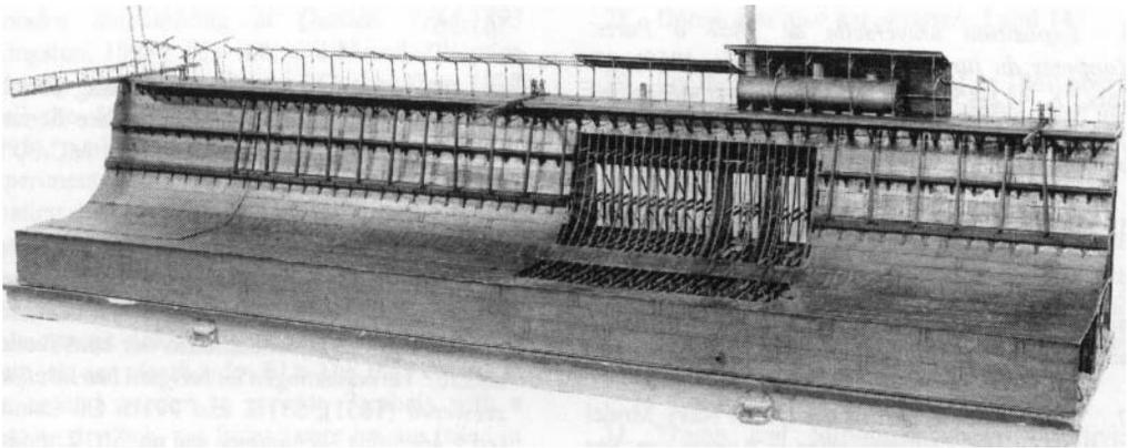
Figure 16: Model of the 1876 floating drydock of Onrust, as yet unrestored.
