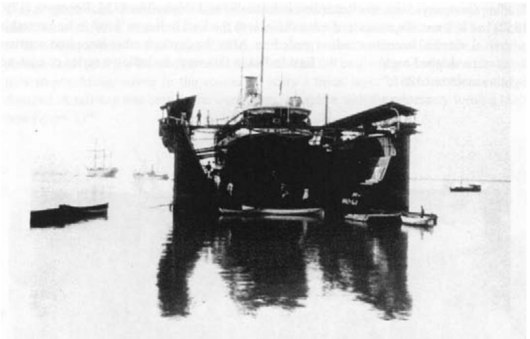
*Figure 5:* A vessel docked in the drydock in Tandjoeng Priok, Batavia harbour.
